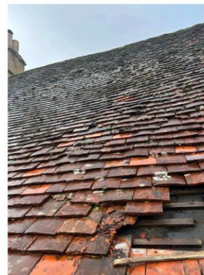
Close up of roof showing delaminated, cracked and missing tiles (photo show eaves being opened up for structural inspection)
